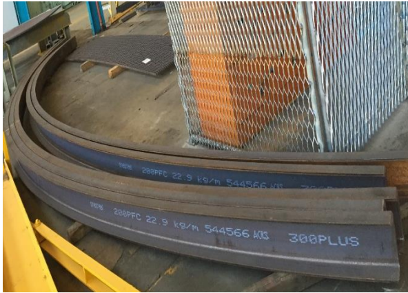
Rolling Structural Steel
